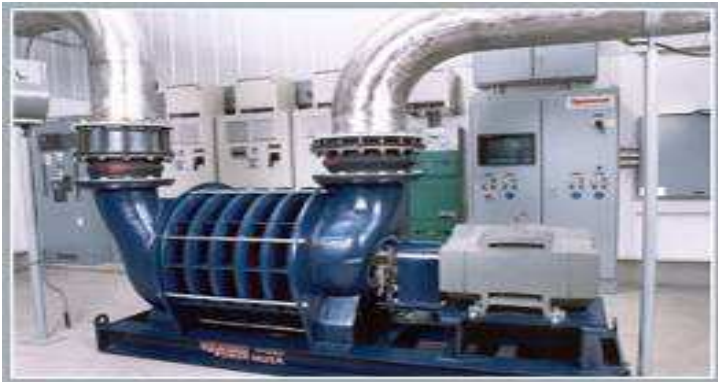
Drinking water distribution ***
