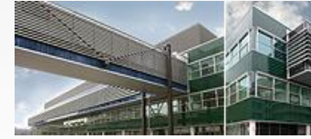
LKH Hospital Steyr, Austria 2 x 20 Gateways
