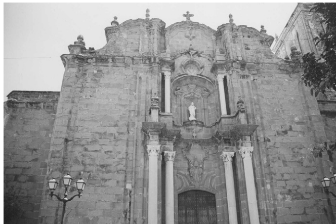
Fig. 1. View of the Puerta del Perdón of the Church of San Mateo in Tarifa.
