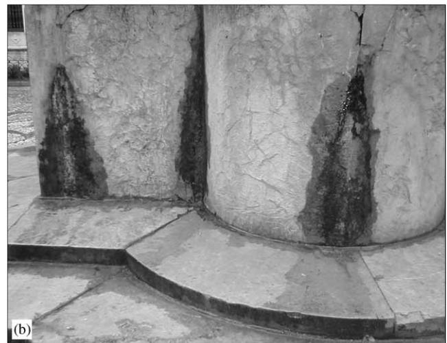
Fig. 2. Effects of biodeterioration: (a) biogenic carbonate crusts and (b) biological patinas on different surfaces of the fountain.
