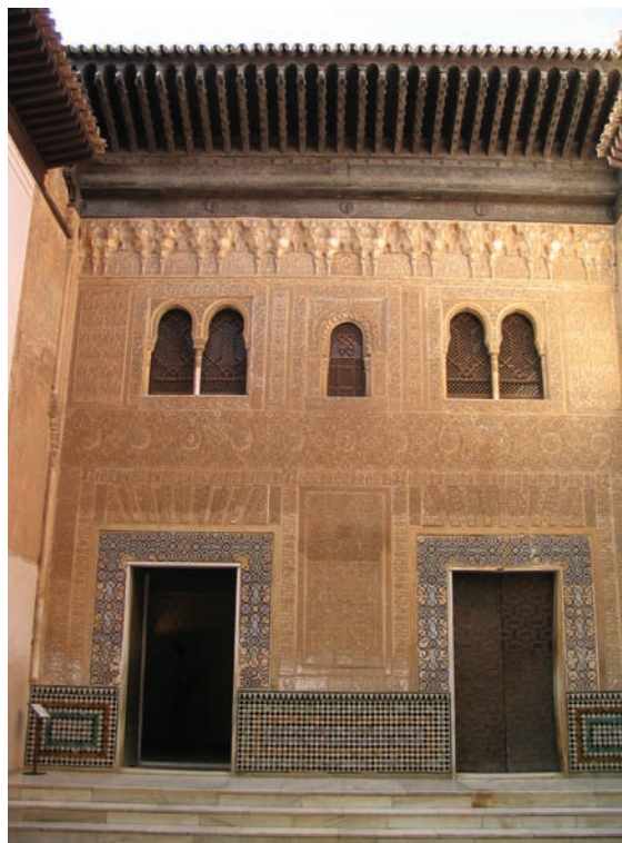
Figure 2 Façade of the Comares Palace showing the basic decoration technique used in the Alhambra: dado tiling at the bottom and stucco decoration above, becoming more intricate with height in the muqarnas. Woodwork is restricted to eaves, doors and ceilings. The eaves of the Comares Façade are considered the apotheosis of Hispano-Muslim carpentry.
