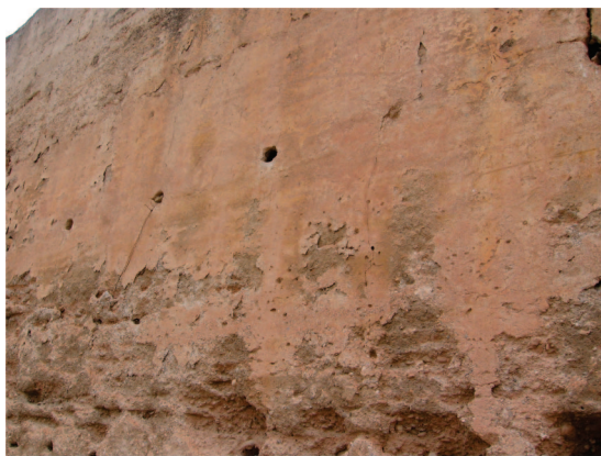
Figure 1. A general view of the 14th century Moorish rampart in the Albayzín quarter of Granada. The circular holes have a 10 cm diameter.
