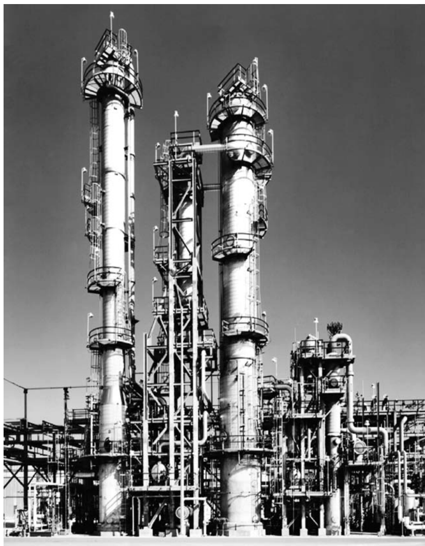
Figure 35. Acetylene recovery plant (name plate capacity: 14 400 t/a of high-purity acetylene)
