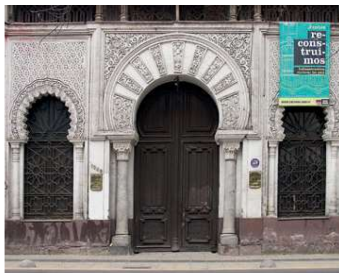
TOP AND LEFT The Palace of the Alhambra in downtown Santiago, Chile, was the first Moorish-style building in Latin America, and it dates from 1862. The work of architect Manuel Aldunate, it was originally a private home. It now houses the National Fine Arts Association. (Map I)
